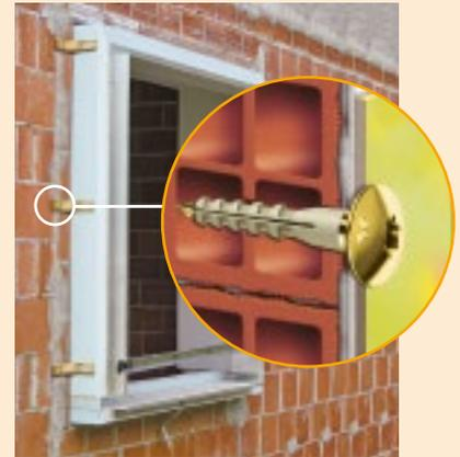
Pose of carpentry with angle bracket.
